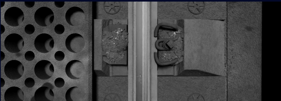
Fixed Track "feste Fahrbahn PORR"
